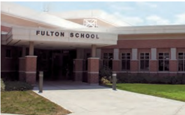
Fulton Elementary School
